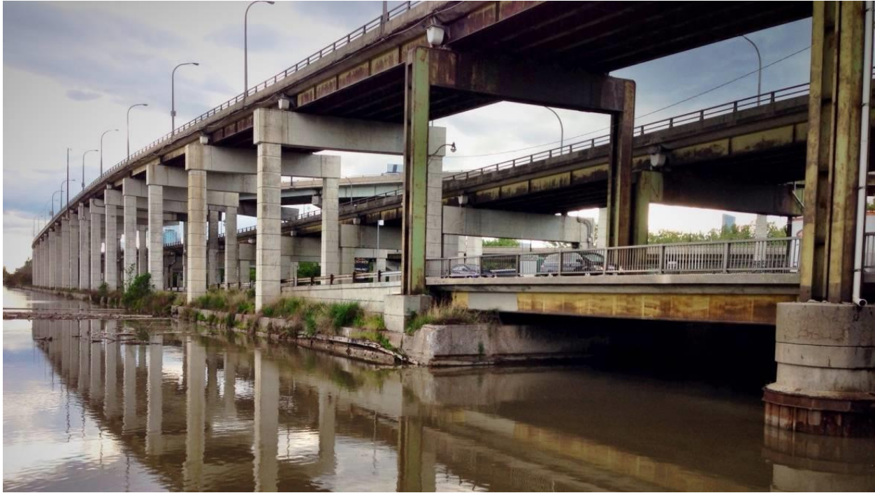
Figure 2. The aging Gardiner Expressway on Toronto's waterfront (Llewellyn, 2016)
