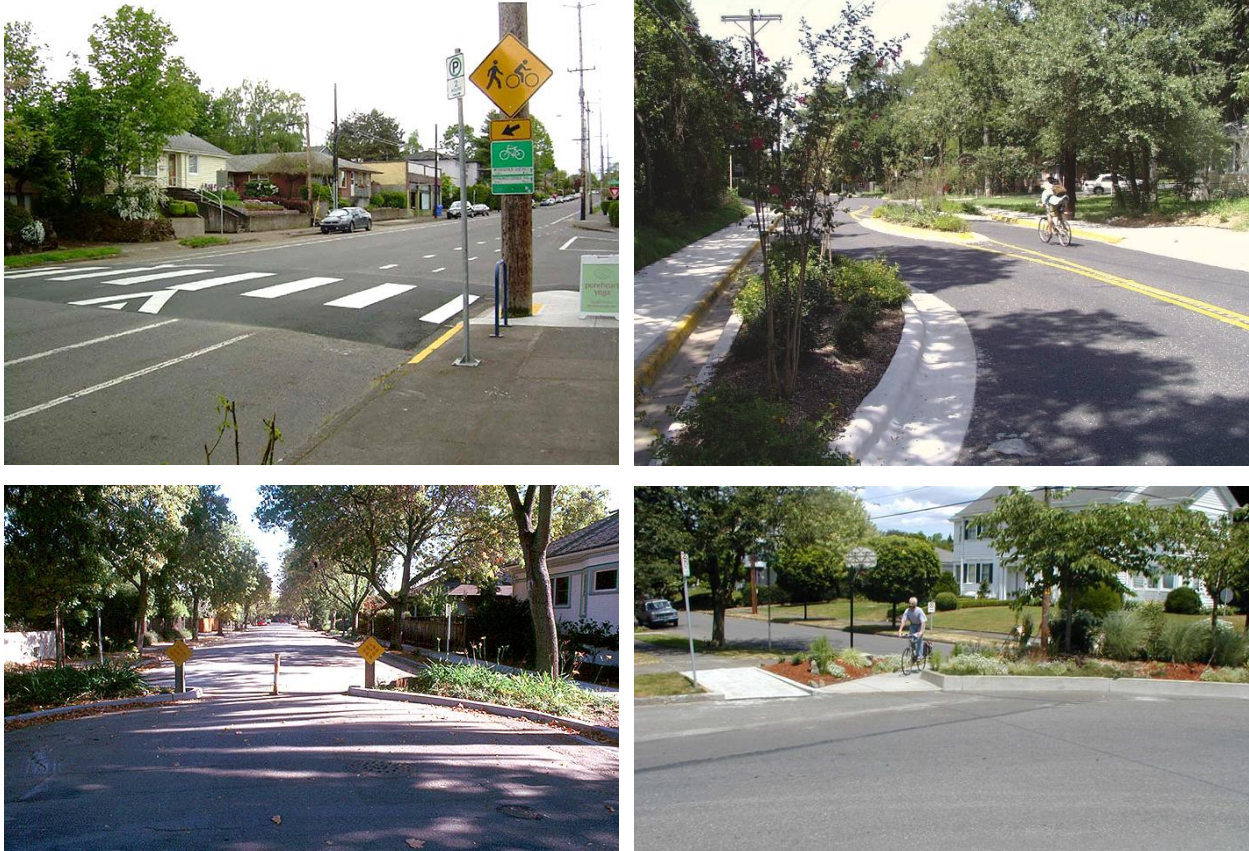
Figure 10. Raised crosswalk (top left), chicanes (top right), mid-block closure with pass-through (bottom left), diverters (bottom right). Sources: U.S. DOT Federal Highway Administration (top left, bottom left), LA DOT Bike Blog (top right), NACTO (bottom right)
