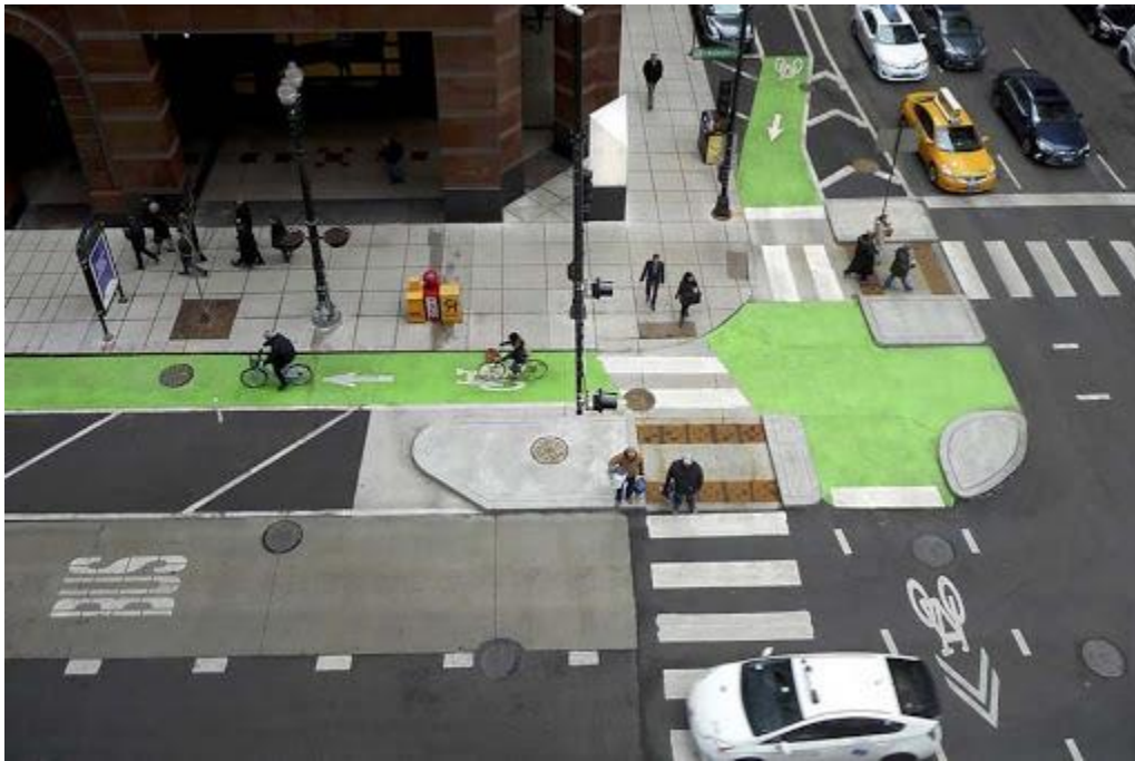
Figure 8. Protected intersection with coloured pavement and elephant feet crossing. Source: City of Long Beach
