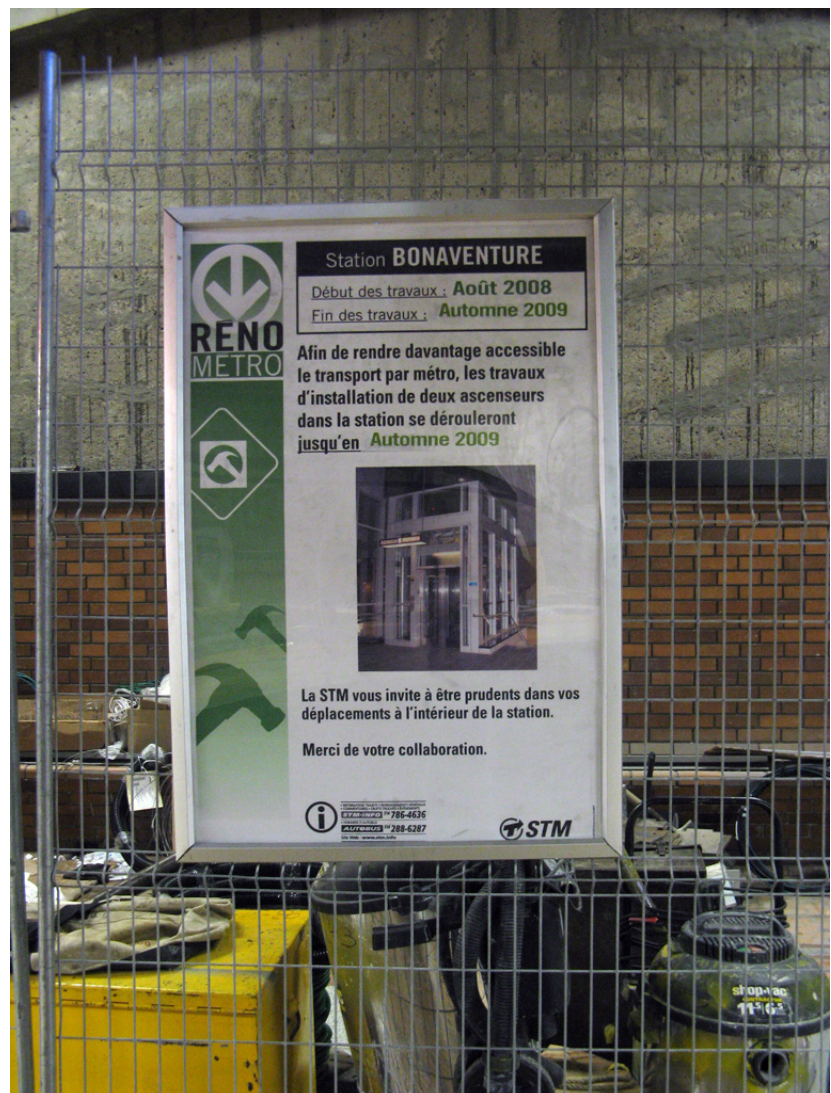
Figure 5: Elevator construction at the Bonaventure Metro Station.
