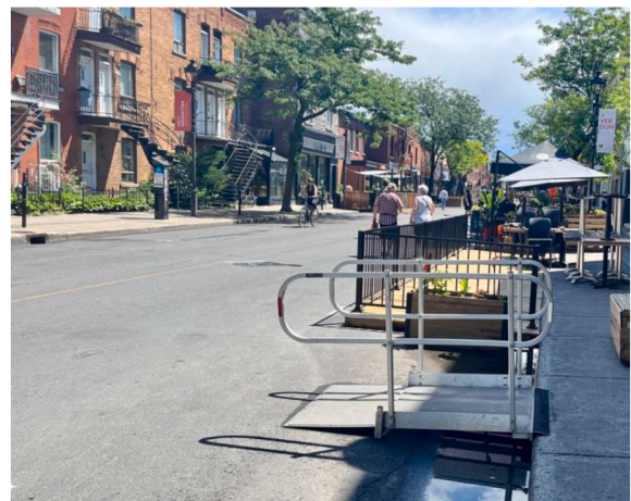
Fig. 3a. Temporary metal accessibility ramp on Wellington Street. Source: Authors.
