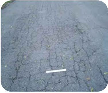
Alligator Cracking
