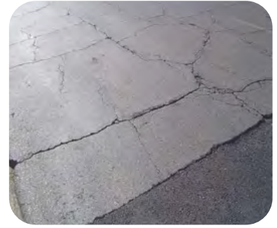
Block Cracking
