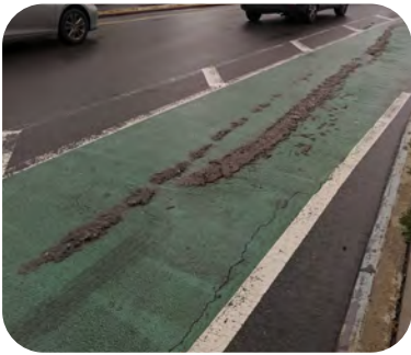
Concrete Spillage
