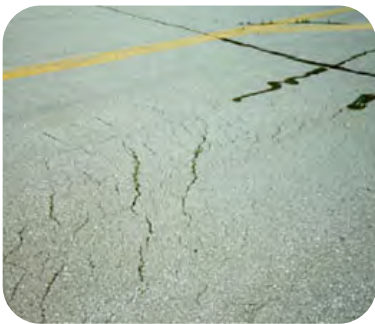
Slippage Cracking
