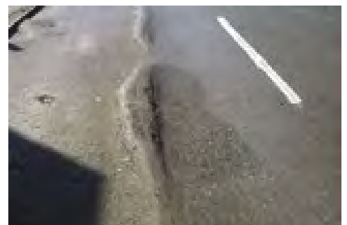
Figure 4 - Pavement Warping
