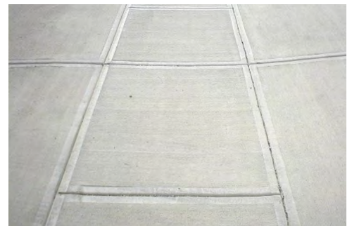
Figure 3 - Concrete Slabs with Joints
